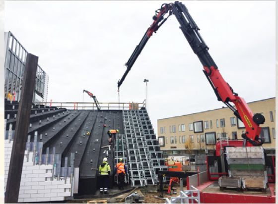
Evolution of the construction site, including the external tiles
